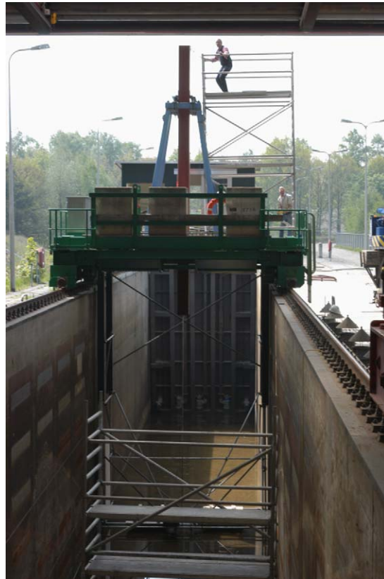
Fig. 3. The vacuum tank (with the riser beneath) mounted on the carriage.
